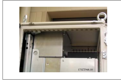
Illustration 3.49: Enclosure top installed
