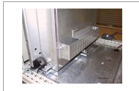
Illustration 3.59: Bottom duct installed.
