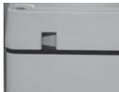
Ventilation holes to prevent condensation
