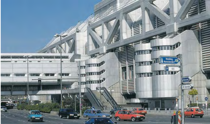
Complex HVAC building services automation solutions
